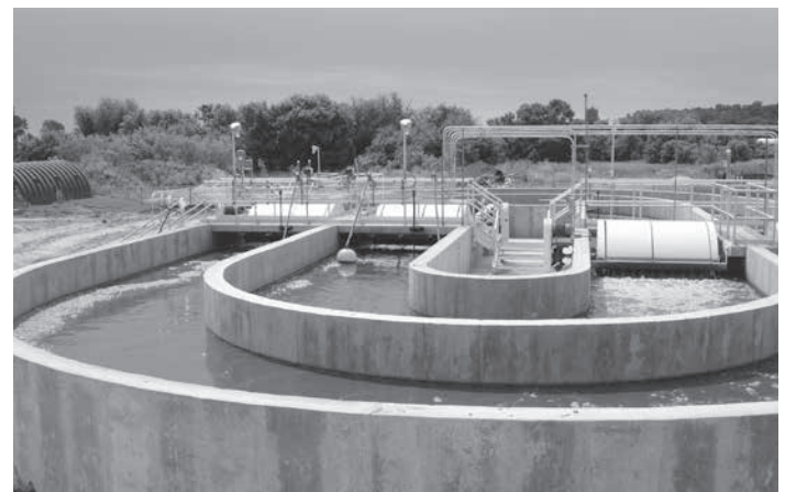
New oxidation ditch
