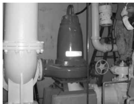
New vertical-mounted dry-pit pump
